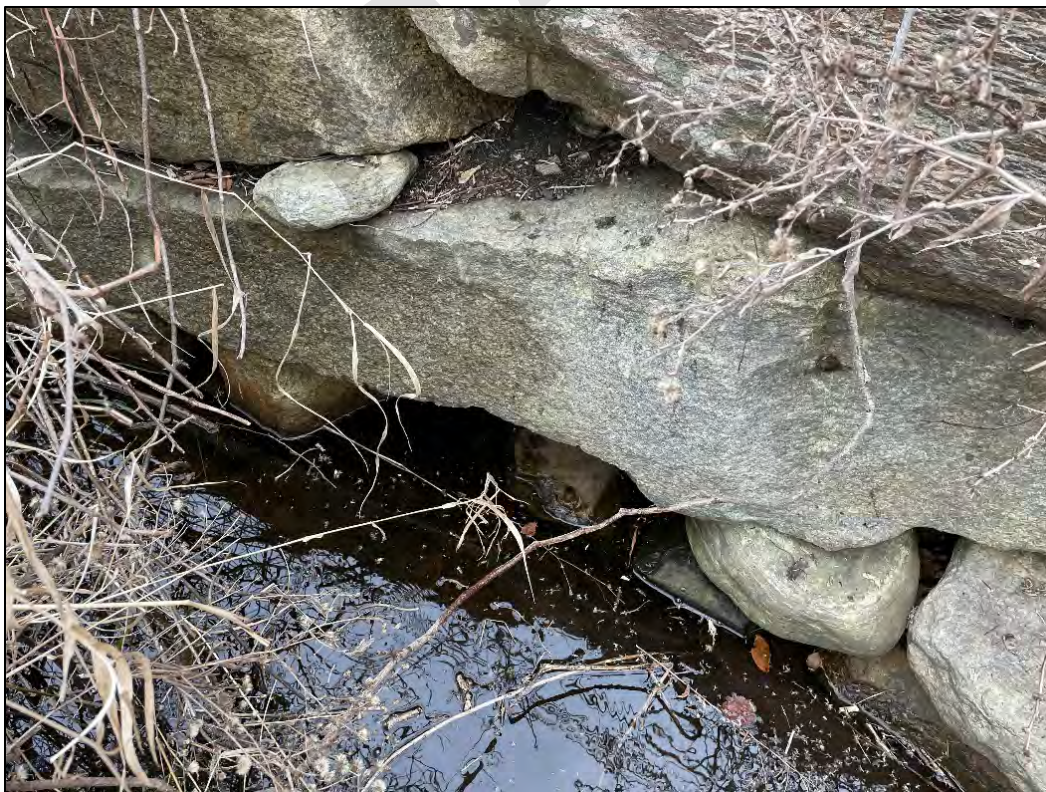
Photo No. 56.: Reach_C_#5.2 - Whitin Road west "culvert" downstream view. No visible culvert; possibly fully collapsed
