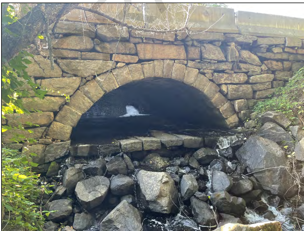
Photo No. 22.: Reach_A_#11.2 – View of the stone arch culvert of the Manchaug Road crossing downstream of Stevens Pond Dam.
