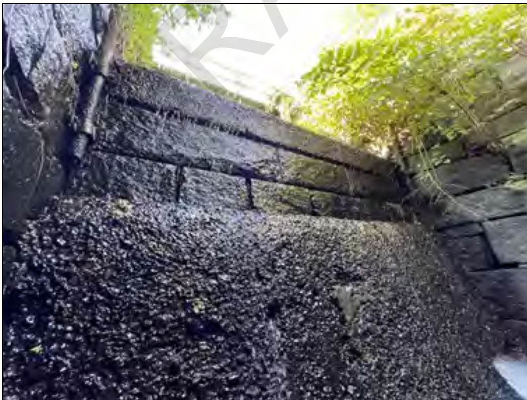
Photo No. 20.: Reach_A_#11.2 - Stevens Pond Dam's spillway. Note the LLO discharging at the base of the spillway (photo bottom right).
