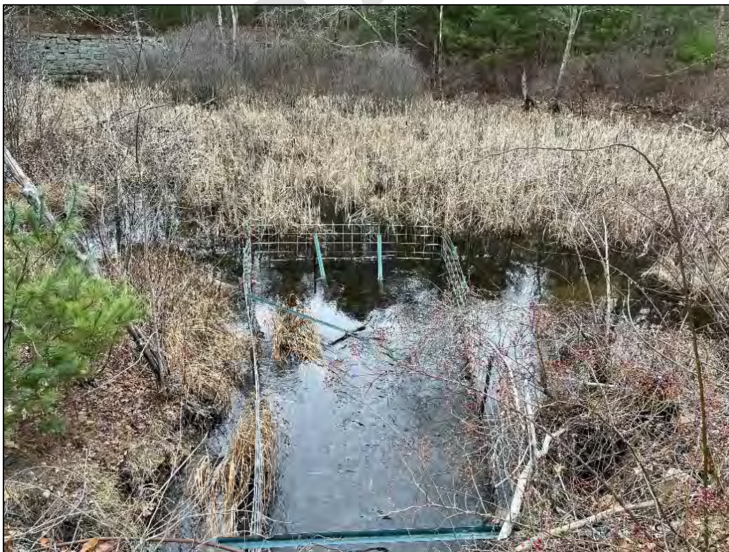
Photo No. 36.: Reach_B_#13 – Beaver decoy installed upstream of the Putnam Hill Road culvert.
