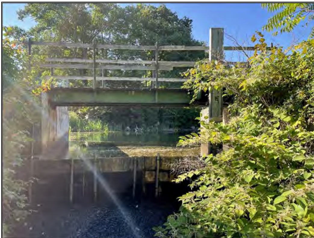
Photo No. 19.: Reach_A_#11.2 - Overview of the Stevens Pond Dam's spillway.
